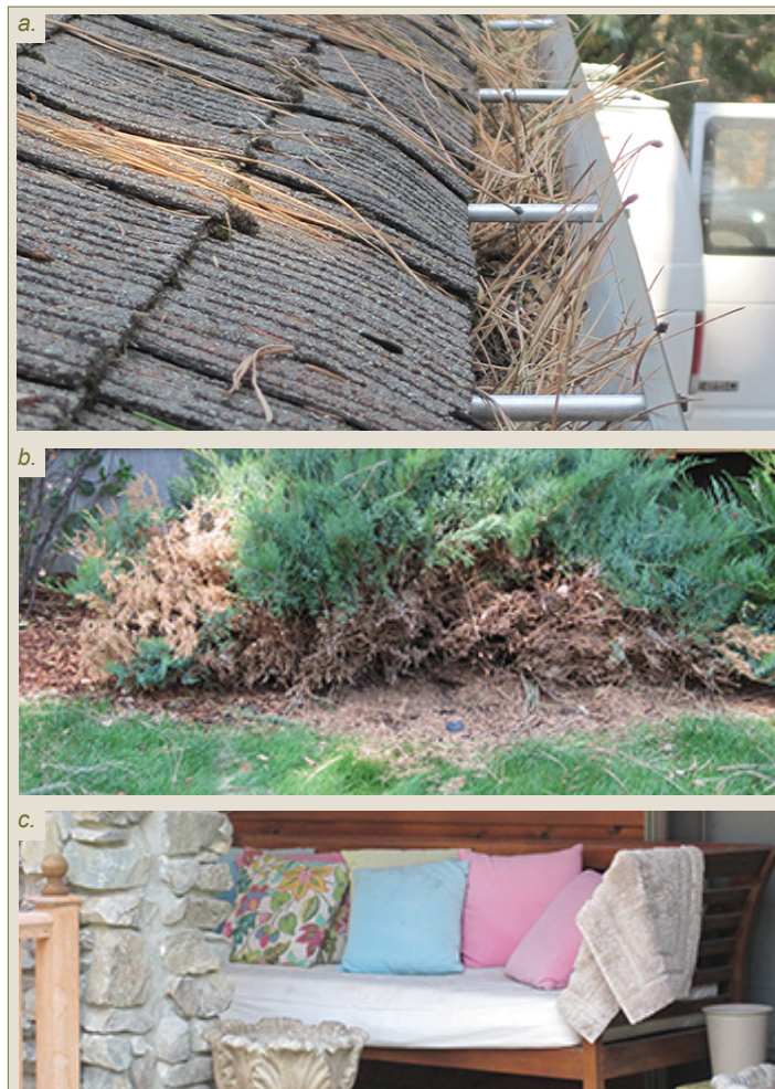
Figure 9. Example firebrand ignition vulnerabilities of houses. a) Burning dead pine needles in the rain gutter can ignite the house at the eave. b) Burning evergreen shrub from ignited dense dead material inside produces structure flame contact on the wall and under the “push-out.” c) Flammable patio furniture cushions and pillows can burn to produce flame contact with the wall and fracture windows that collapse to allow firebrands and flames to penetrate the interior.
